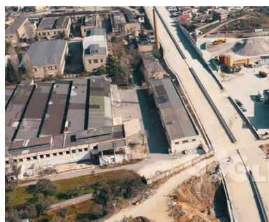
Fig. 4. "Traktore" Plant, Drone View 2021
