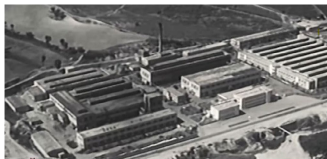
Fig. 3. "Traktore" Plant, Air View 1965
