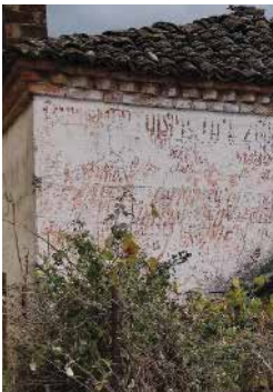
Fig 9/ Typical construction techniques: on the left stone masonry with wood strips; in the center adobe masonry; in the right plastered stone masonry with brick mouldings and terracotta roof tiles. — source/ author (Pustec 2023)
