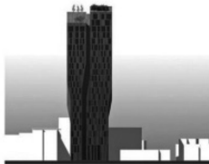
All concrete walls – No columns due to Challenge & Individuality
