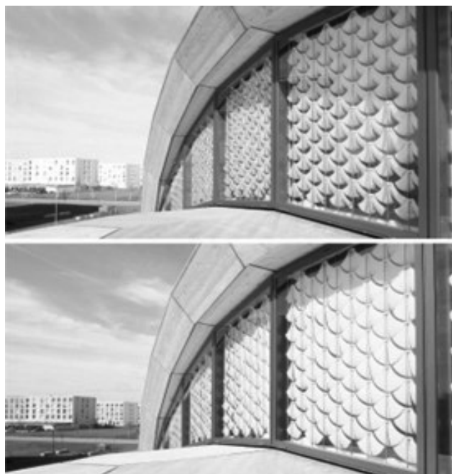
Figure 4. The 4D-printed shading elements open to let in sunlight during a cool morning (top) and close to block heat during a warm afternoon. (Image © Tiffany Cheng, ICD University of Stuttgart)
