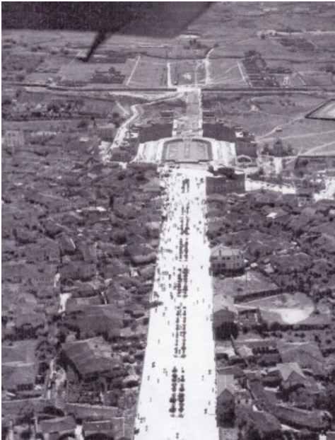
In Figure 18; Aerial View of the Spine, 1940.
