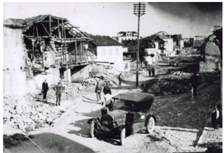
Fig. 6, View of the destructions caused from the 1926 earthquake in the Castle district
