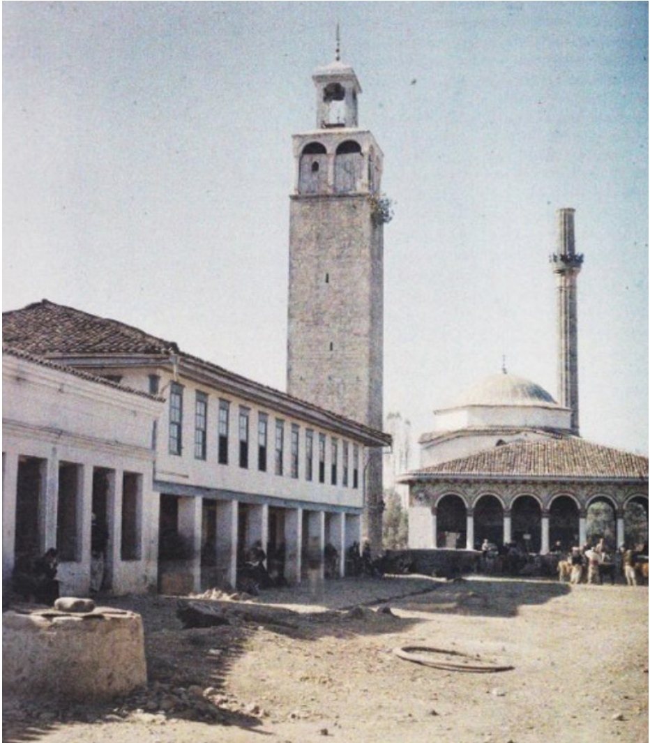
In Figure 5; The Ethem Beu Mosque. Minaret with missing roof (1913)
