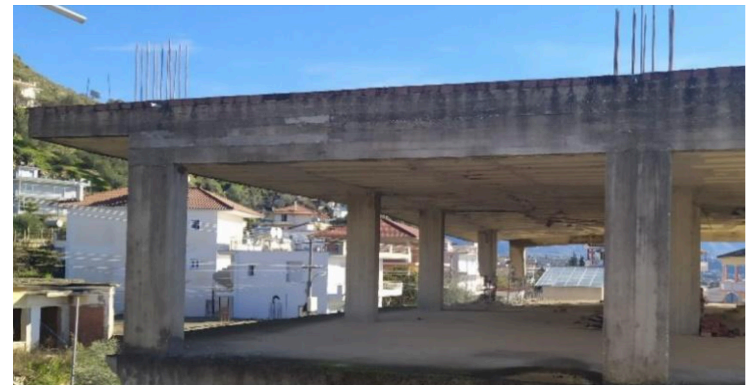
Fig3 / Wall case study: a) top view of Finiq and location of the building considered [21] b) lateral view of the specific façade of the building considered. source / the author
