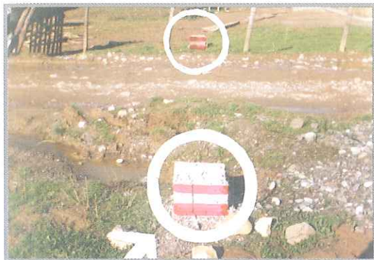
Pointing on site of the future public spaces and roads
