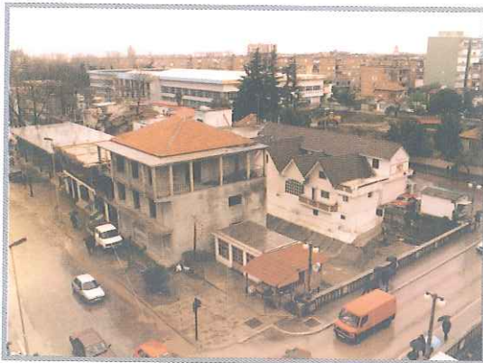
View of illegal construction and kiosks over Lana river
