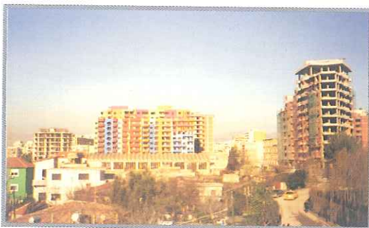
Flat buildings on construction near Park of Tirana, January 2003
