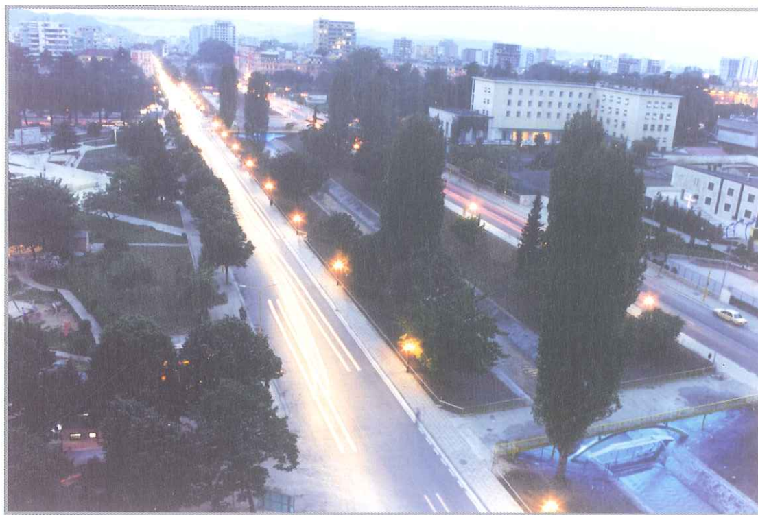
View of refurbished road along Lana river
