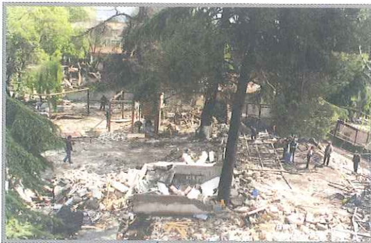
Demolition of kiosks in the Park "Rinia-Youth"
