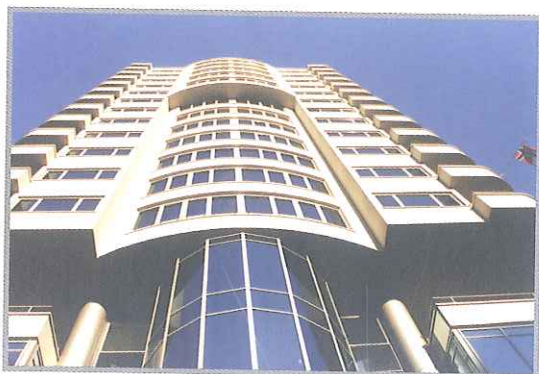
Sky Tower, built on year 2000, one of the new modern symbols of business and financial centers
