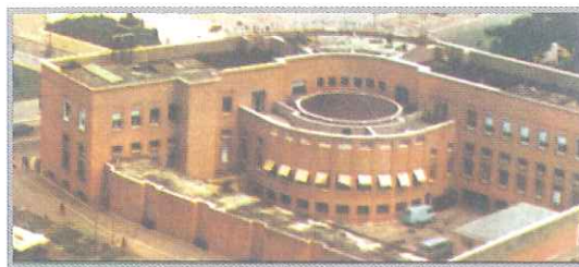
View of the rear part of the National Bank built on 1930-38
