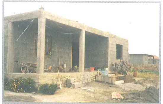
Building the first floor
