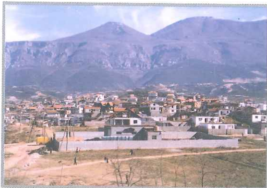
Illegal construction in north – east of Tirana
