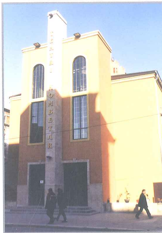
Refurbished front view of the building of National Theatre located in the centre of Tirana
