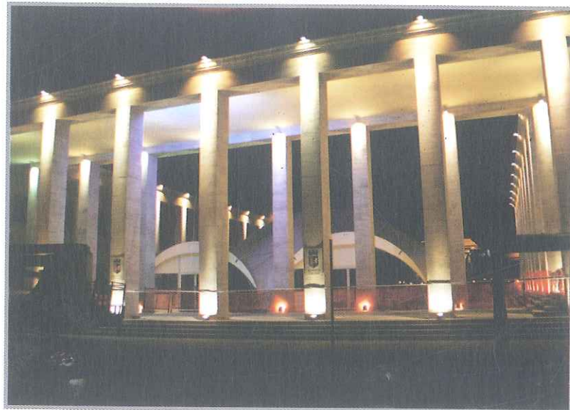
New pavements and lightings
