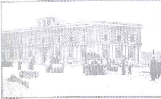
The finishing works of Scanderbeg Square, in the front: former Ministry of Internal Affairs.
