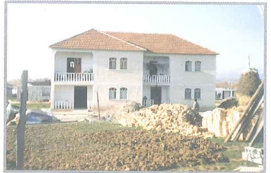
Completing the house
