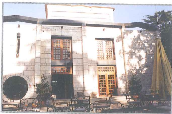
Refurbishment of the building of Cinema "Millennium 2" constructed on 2001 in the side of the walls of Toptani castle-house
