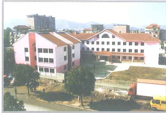
Reconstruction of eight year elementary school "Sabaudin Gabrani" located in the west part of the ring of Tirana funded by OSFA Soros Foundation
