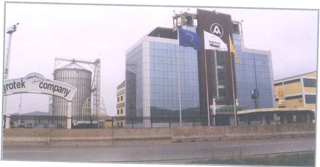
New industrial buildings
