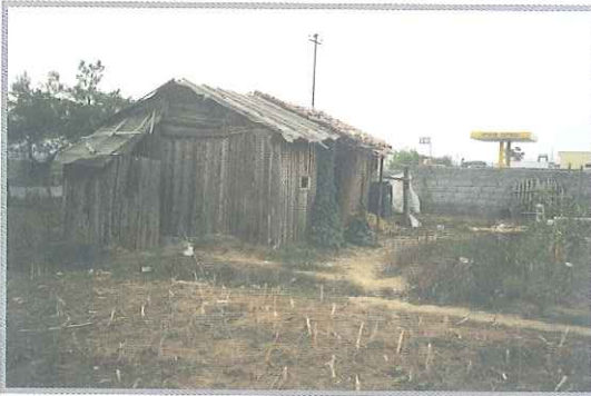
Building a "barrake"
