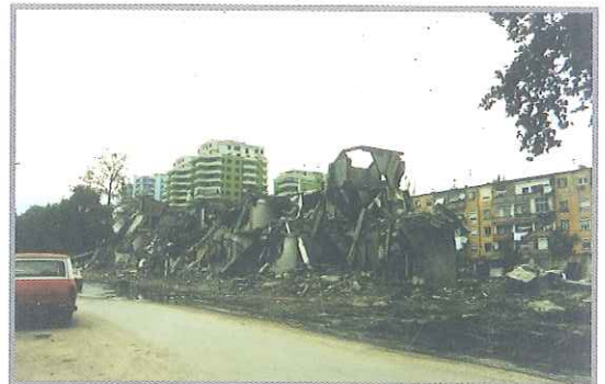
Demolition of kiosks in the banks of Lana
