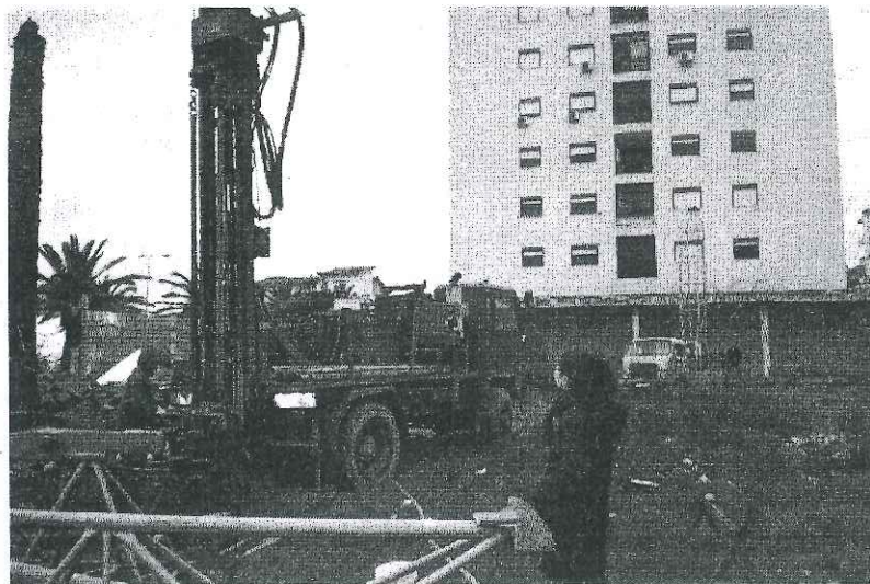
Fig. 1. Its show view of a geotechnical investigation closed to former building
