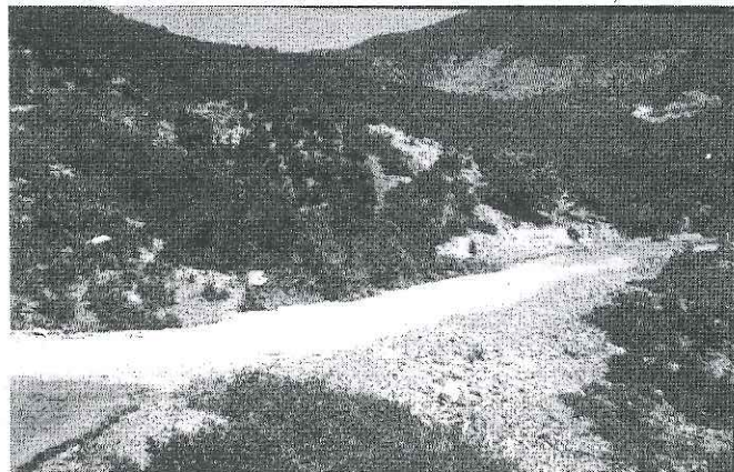
Fig. 10. Shkopeti landslide. It's looking to north-east, and shows, the movement of Miloti-Burreli road filled by gravels and landslide body
