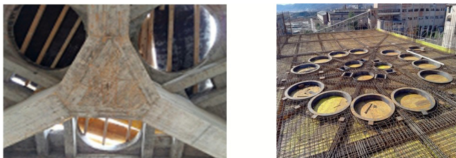
Fig 2. The connection between concrete slabs and silos, some details.
