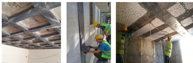
Fig 5. Photos of the building during construction works
