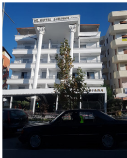
Fig 4. Lubjana Hotel after the earthquake of 26 November (Source: Klodjan Dervishi)
