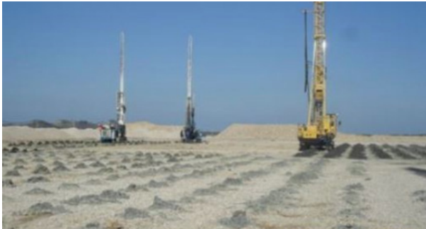
Fig 6. Drilling of boreholes for vertical drainage system (Source: Luljeta Bozo)
