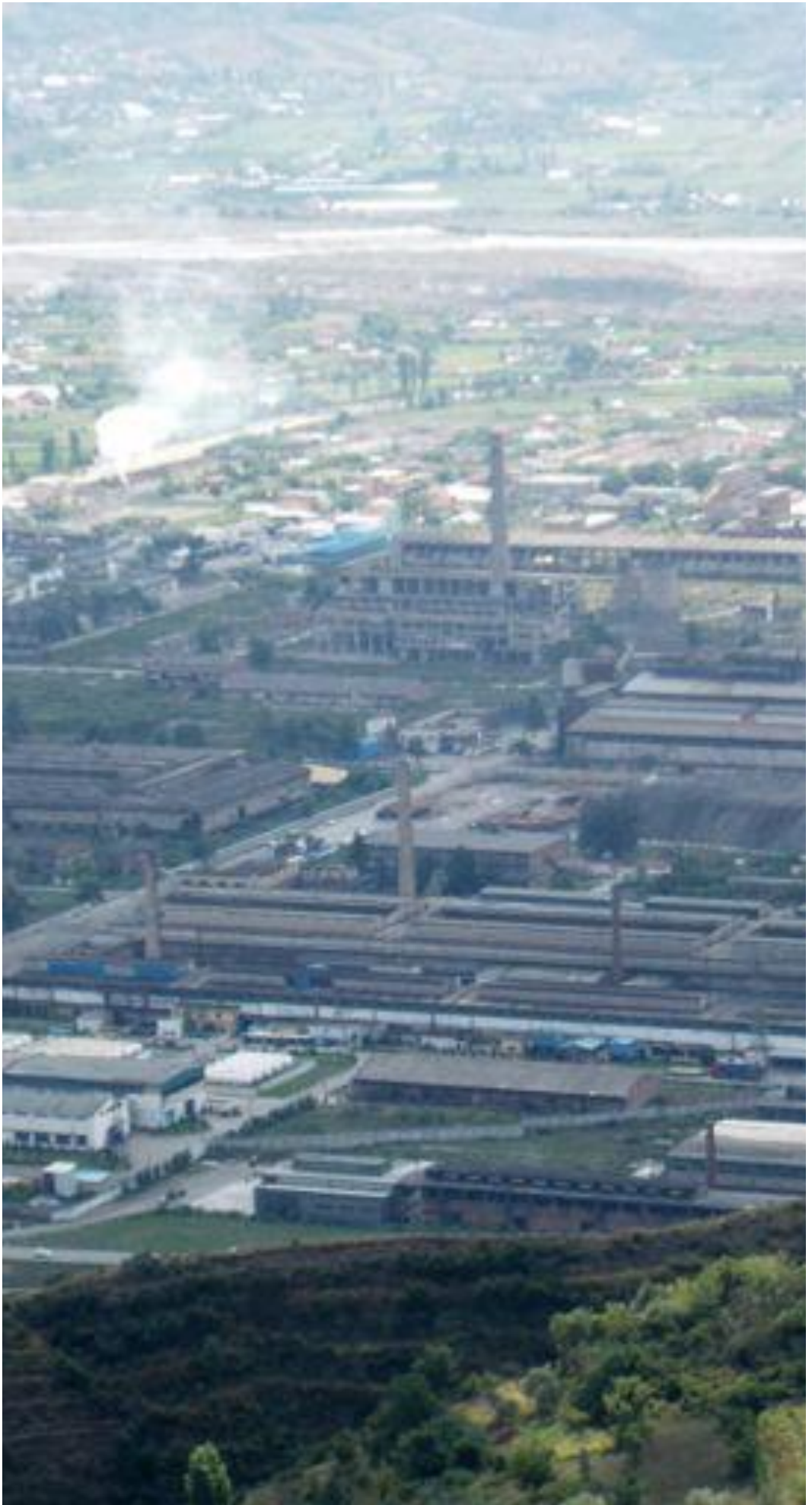
Fig2 / aerial view of the Elbasan metallurgical complex built in 1974 and called the "Steel of the Party" source / internet
