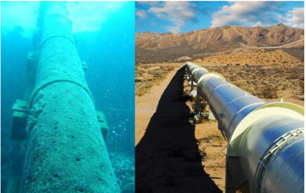
Fig3 / the Trans-Adriatic Pipeline (TAP), under construction, will connect with the Trans Anatolian Pipeline (TANAP) at the Turkish-Greek border at Kipoi, cross Greece and Albania and the Adriatic Sea, before coming ashore in Southern Italy / source internet
