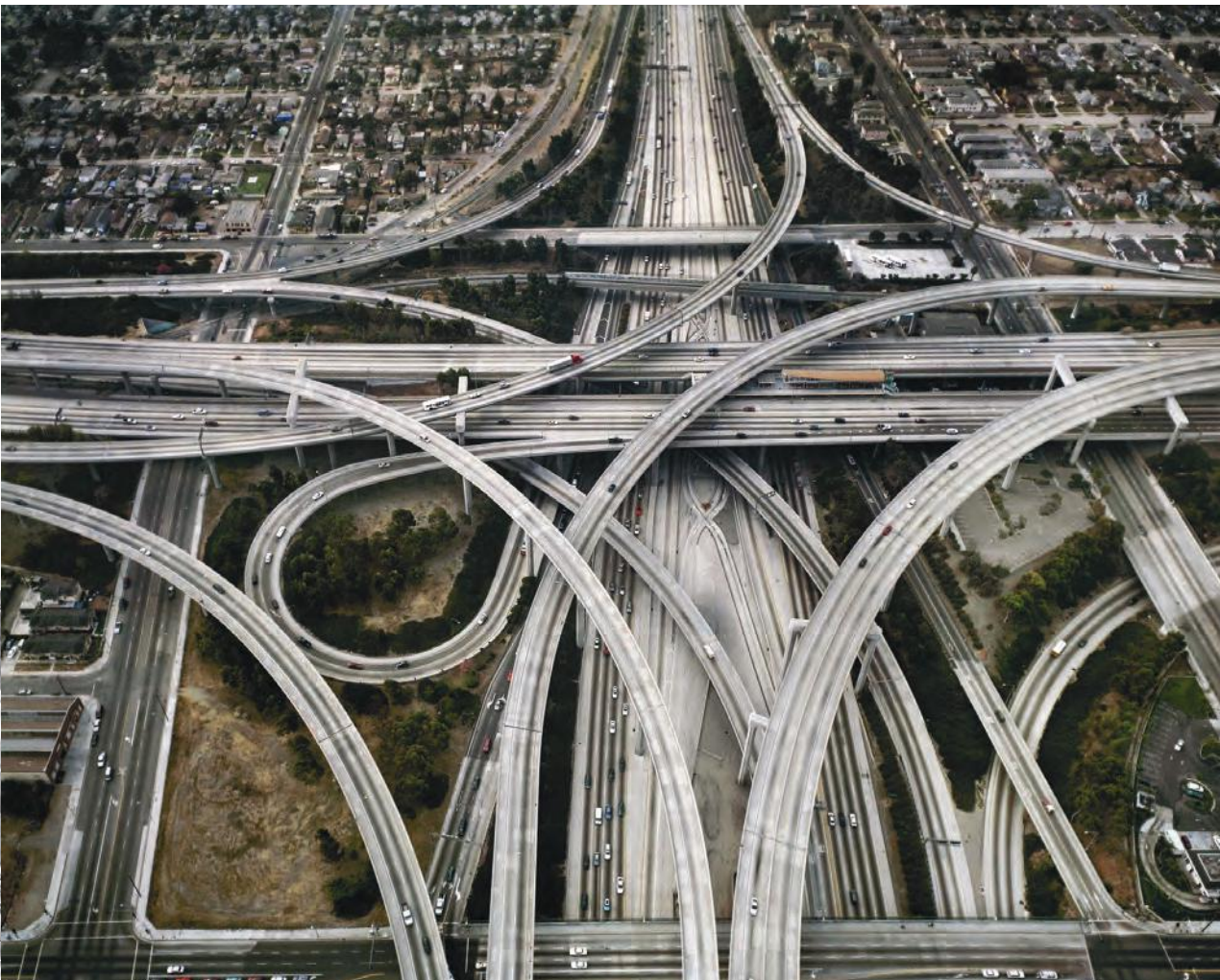
Fig. 2. Motorways, Los Angeles '70
