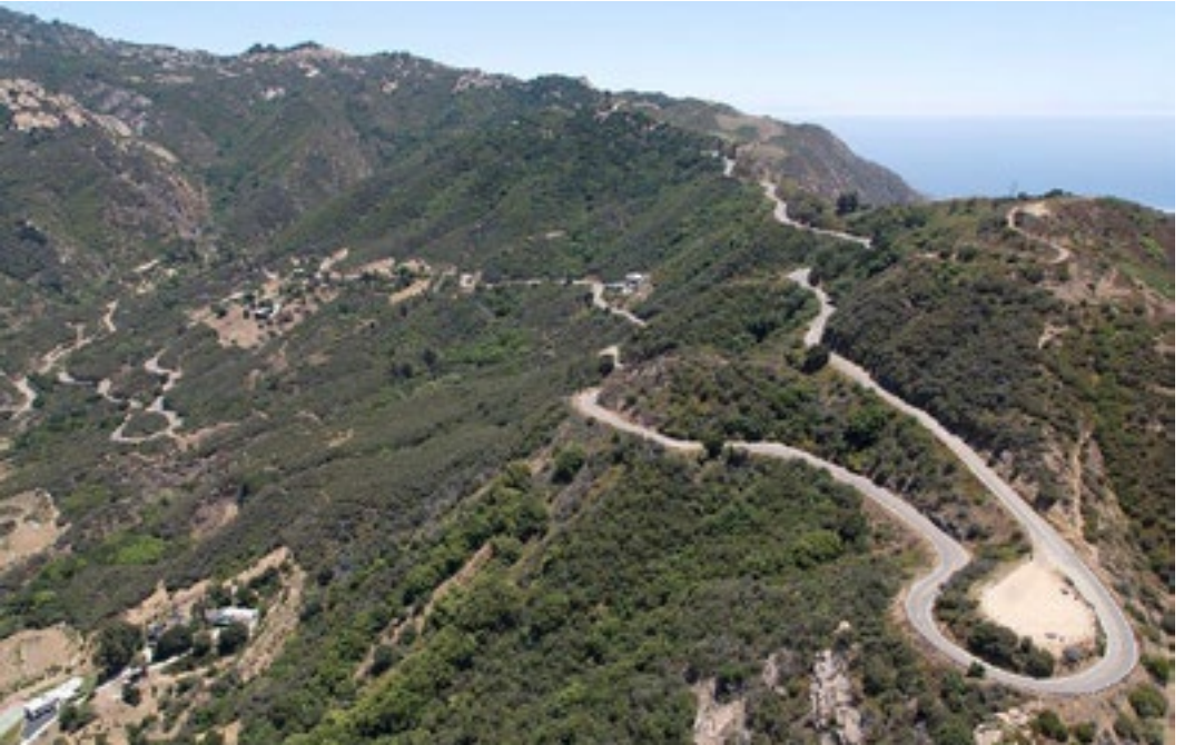
Fig9 / The sharp curves along Mulholland Drive, Los Angeles, CA source / internet
