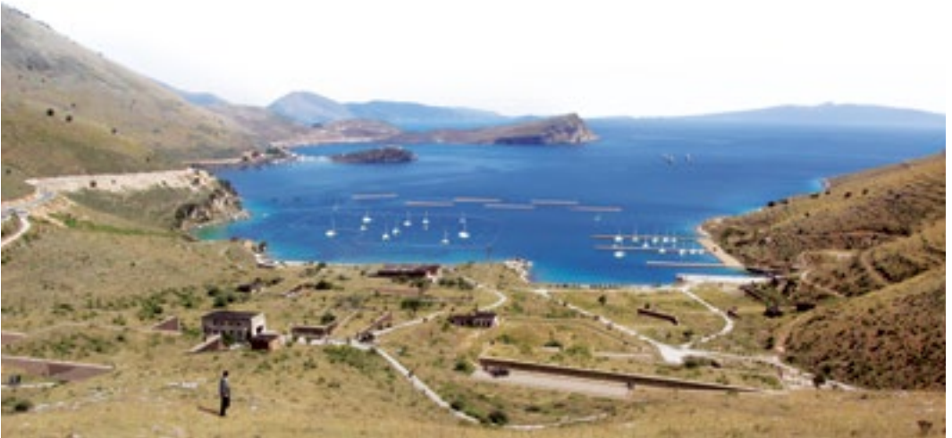
Fig1 / Rendering of the project "Reactive Riviera," source / Re-Active Riviera competition panels Source: Metropolis, Sealine.
