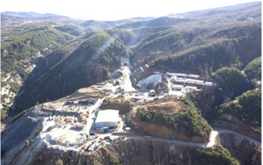
Fig 1 / the New Highway Tirana - Elbasan under construction from KLM 2+850 (distance counting starting from Tirana) up to the Entrance of the Krabe Tunnel KLM 15+650 / source AKTOR
