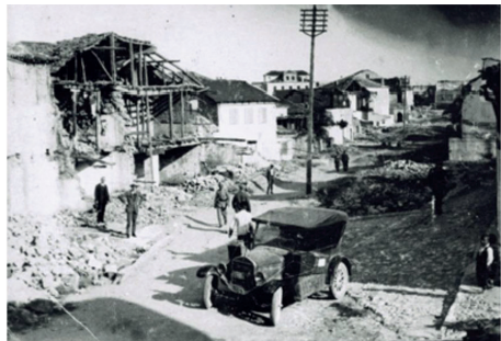
Fig. 6, View of the destructions caused from the 1926 earthquake in the Castle district
