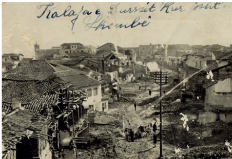
Fig. 5, View of the destructions caused from the 1926 earthquake
