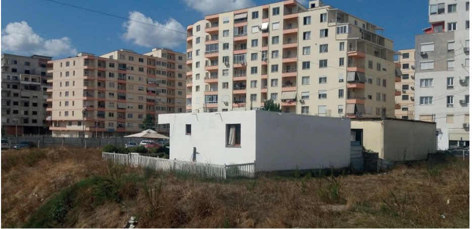
Figure 3 Kashar area, two different housing typologies inside the same urban block. (font: Picture by the author).
