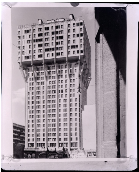
Figure 2. Torre Velasca Milano Designed by BBPR 19250 (Source: Photo by Paolo Monti in 1973)
