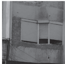
EXTRA SPACE-STORAGE AREA
