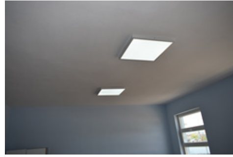
Fig. 5 Interior of the classroom with new lighting fixtures. Source: the author
