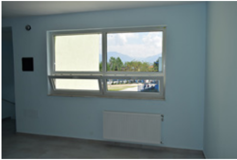
Fig. 4 New double-glazing windows and new radiator. Source: the author
