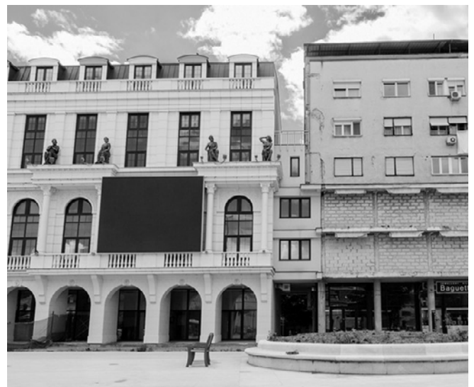
Fig. 21 Unfinished project hew facade Source: photo Peter Nientied, 2019
