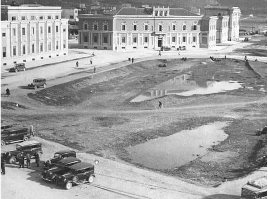
Figure 3: Skënderbej Square under construction during the 30-s. Source: Polis University Archive
