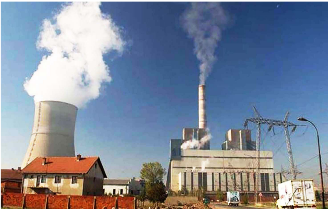
Fig1 / Obiliq Power Plant Source / www.insajderi.com
