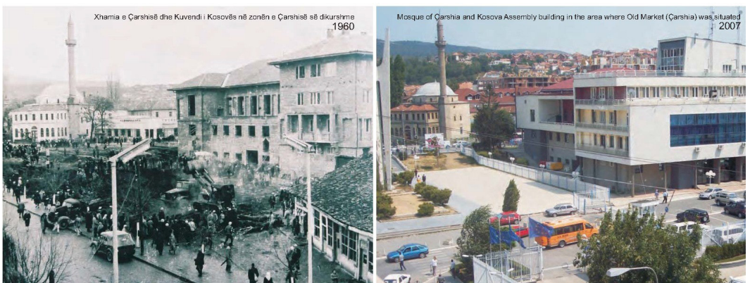
Fig3 / Two pictures: Demolition of Prishtina bazaar and actual situation - Brotherhood and Unity square (1960). Source / Prishtina Municipal Archive)
