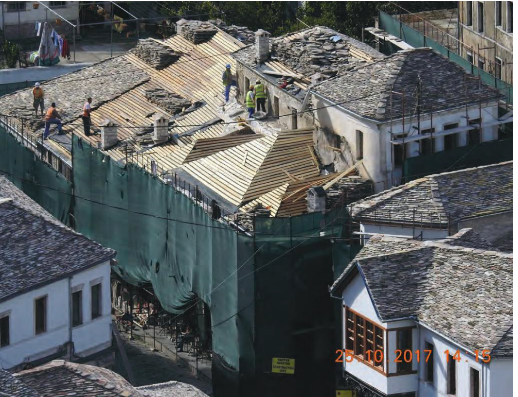
Fig 6 / Restauration Process at TID Gjirokastra Bazaar. Source / Albanian-American Development Foundation
