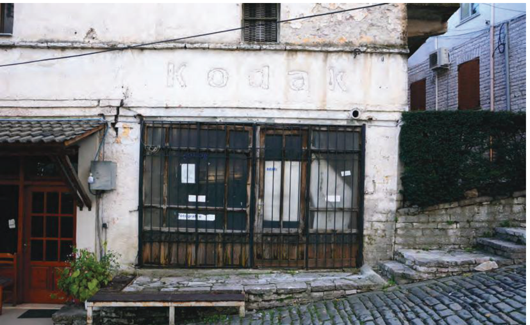
Fig. 3 / Abandoned Shop in Gjirokastra city. Source / the author
