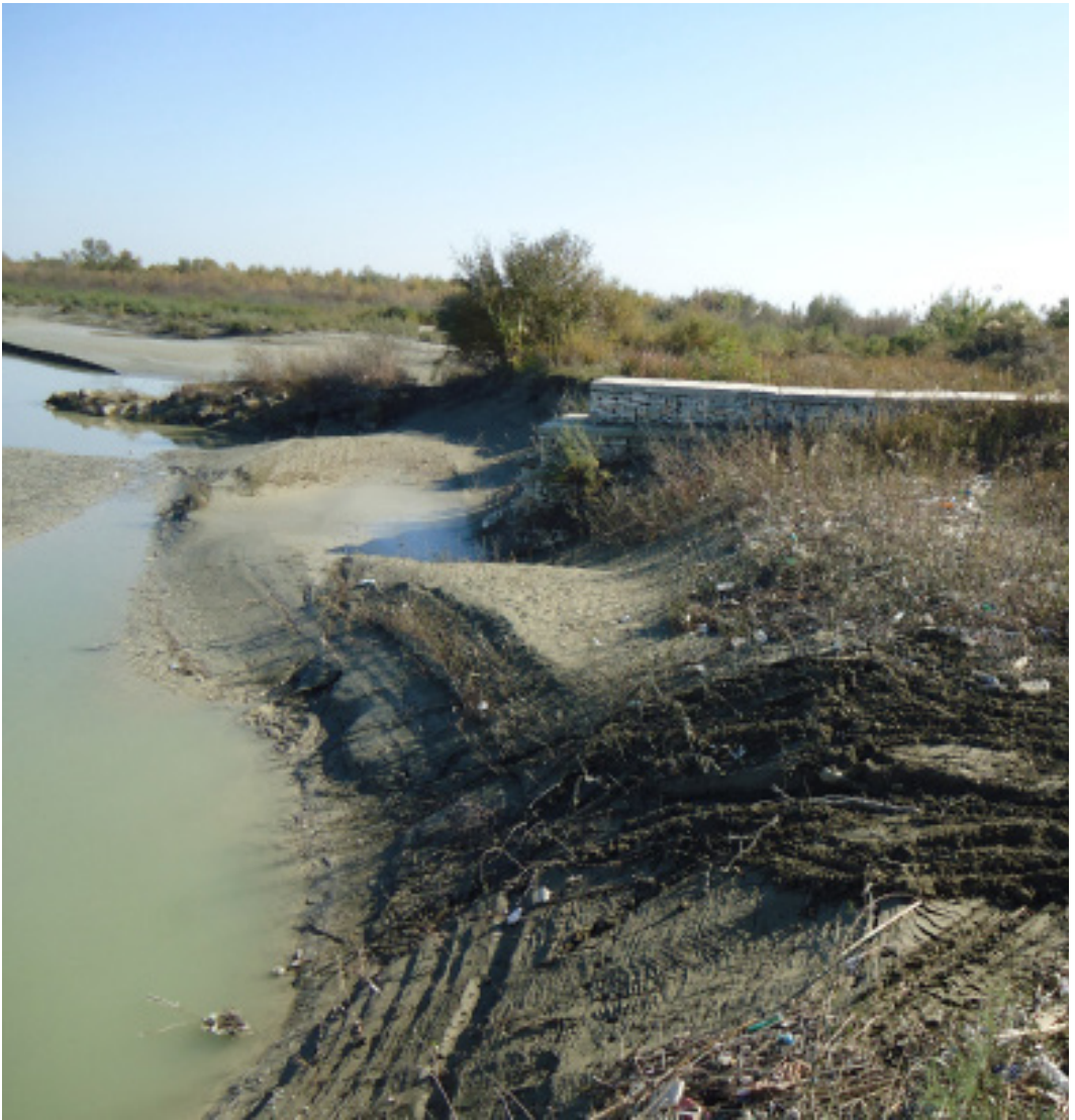
Fig6 / Constuction for Semani riverbank protection source / the author
