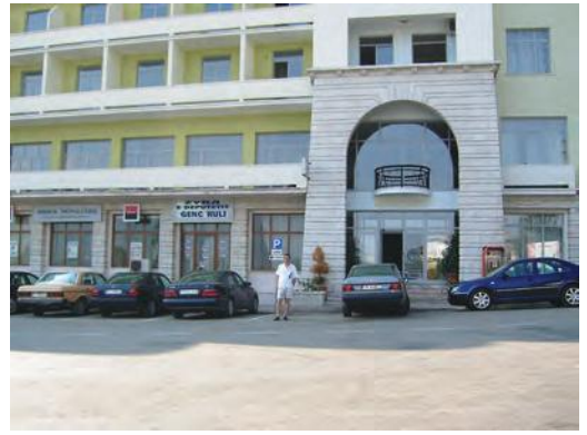
Fig. 16 / View of the "Çajupi" Hotel, Entrance Detail. Source / the author.
