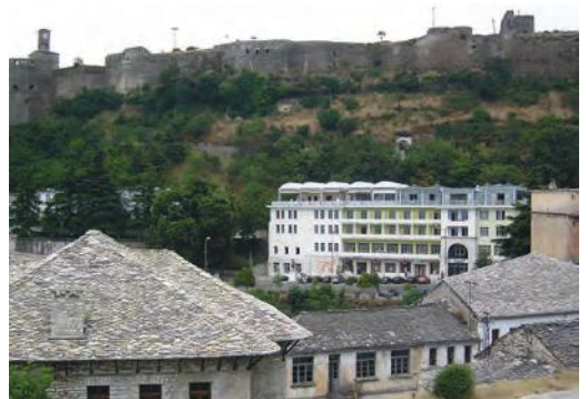
Fig. 13 / Panoramic View of the "Çajupi" Hotel from the Court's Hill (Photo by author).
