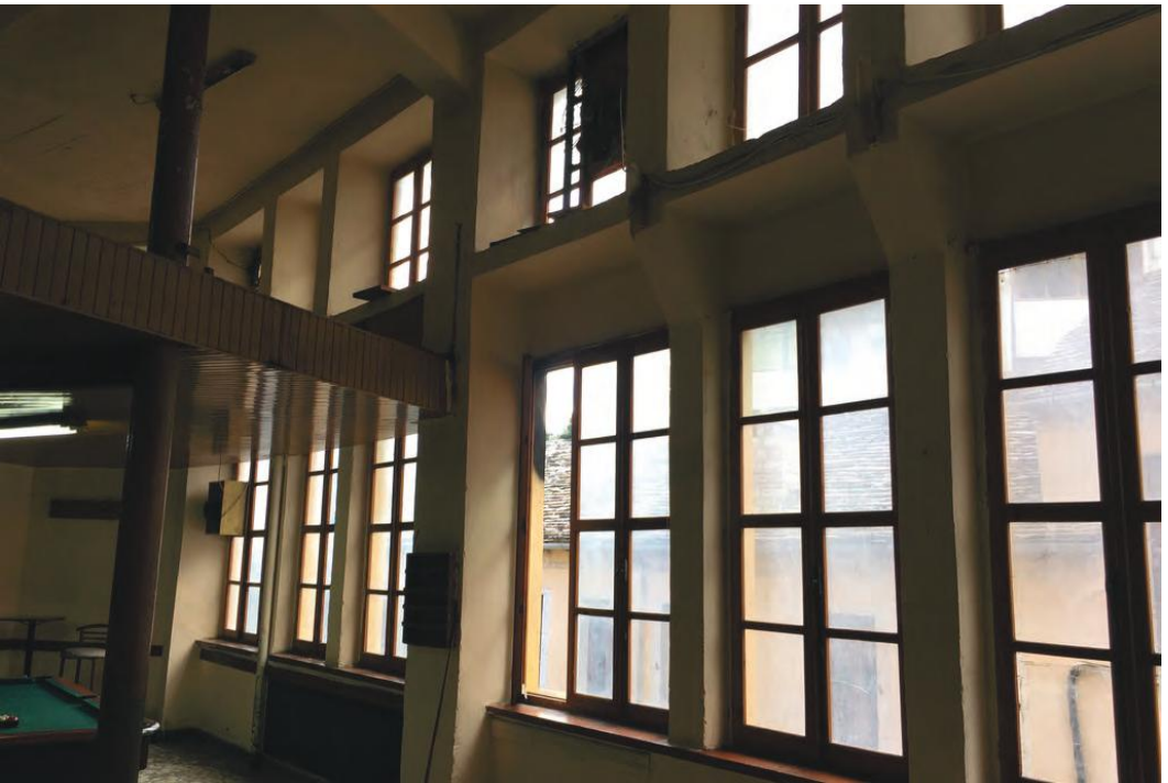
Fig. 6 / Zigai's House, Interior view of the fenestration and the concrete structure.
