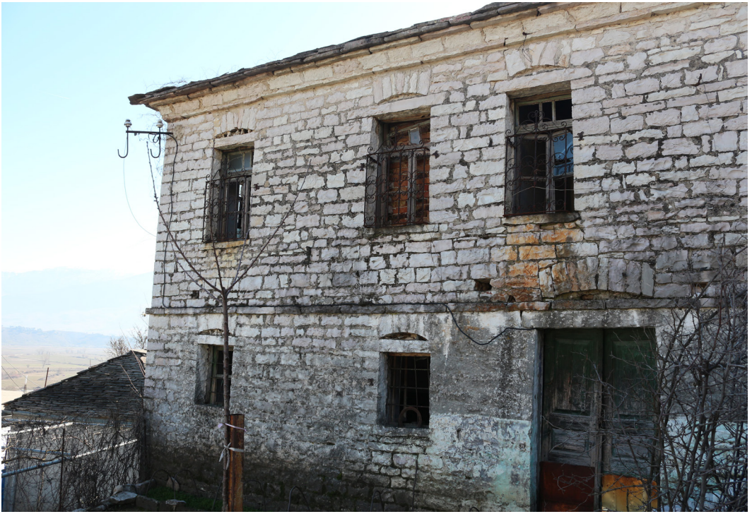
Fig. 1 / Traditional stone house on Dervician, the selected building (February 09, 2019) Source / the author
