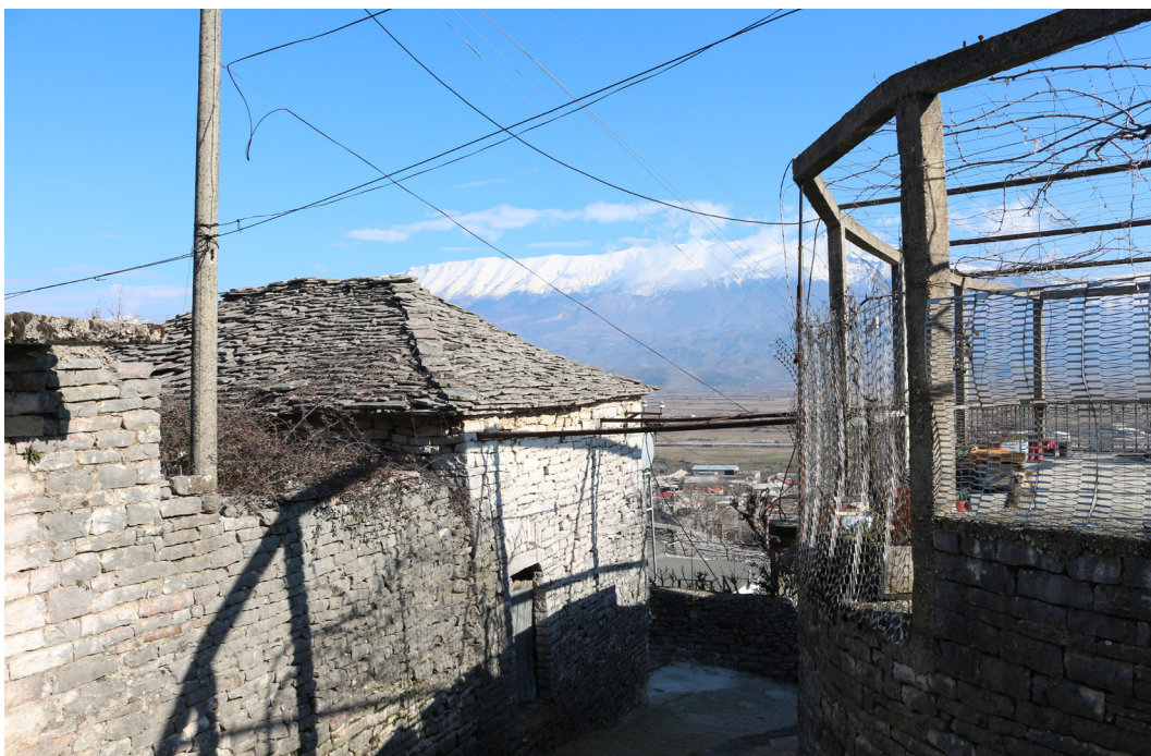
Fig.4 / Example of wrong intervention in the cultural heritage of Dervişan: concrete elements replace ancient structure ignoring one of the restoration principles, the material compatibility. Source / the author.
