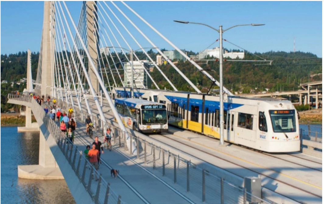
Fig5 / Multimodal bridge in Portland, Oregon is an example of a transformational investment that supports a low-carbon and resilient city / source: City of Portland
