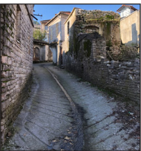
Remove the concrete paving and restore the cobblestones
