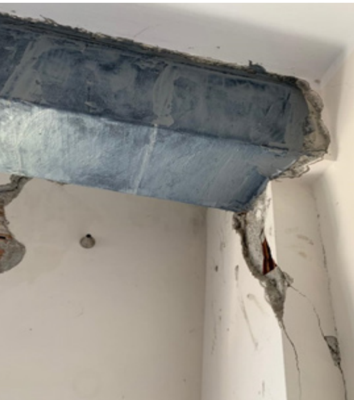
a) Structural damage in the beam b) FRP reinforcement in the beam c) close-up view of the reinforcement d) non-structural damage (partition walls)
