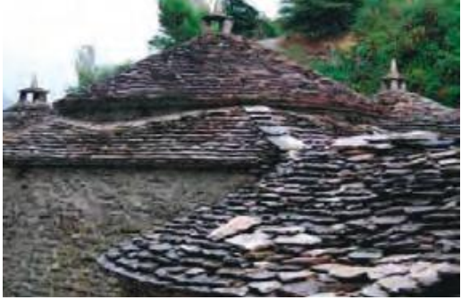
Stone roof of the Hamam
