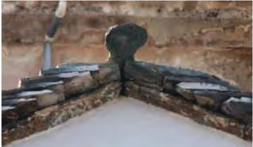
Stone roof detail
