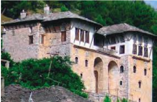
Gjirokastrian residential building
