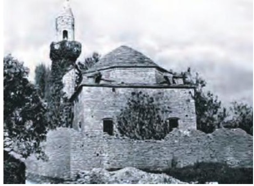
Just as fountains could have their origin in the Vakf the mosques and madrasas could. To the left, a now disappeared, beautiful mosque in the Manal-at block.
