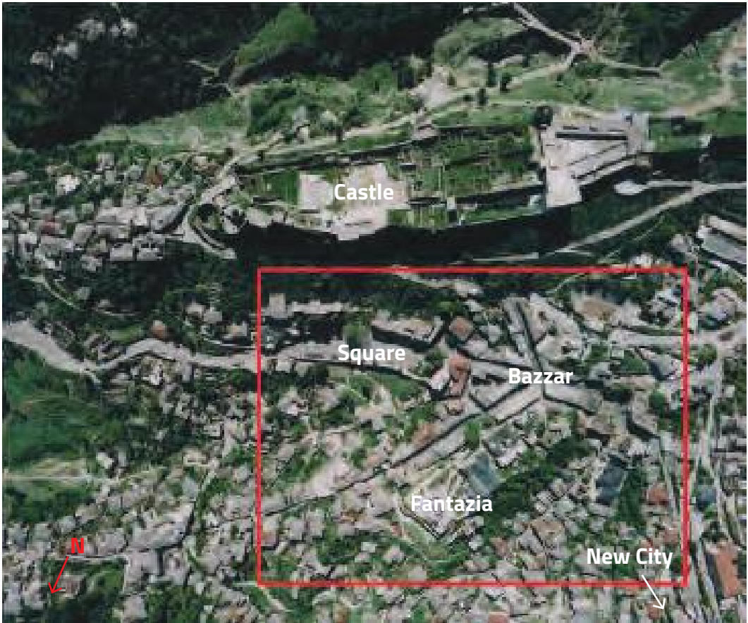
Old Town of Gjirokastra from above, studied area marked with frame.
