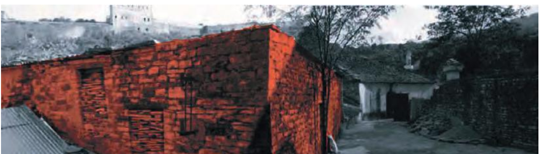
Panorama photo collage of Babameto Building and the yard - view from the north
