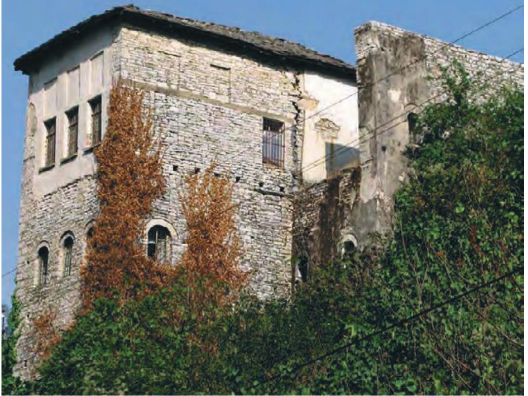
A common view in Gjirokastra, the impressive walls of cut limestone with symmetrical windows and heavy stone roof. Photographer: Elsa Notstrand
