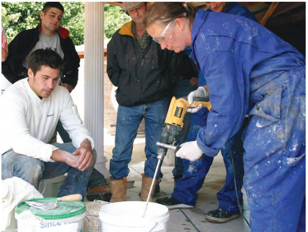
Scottish craftsmen mixing mortar together in the Scottish Lime Centre. Photographer: Roz Artis Young
