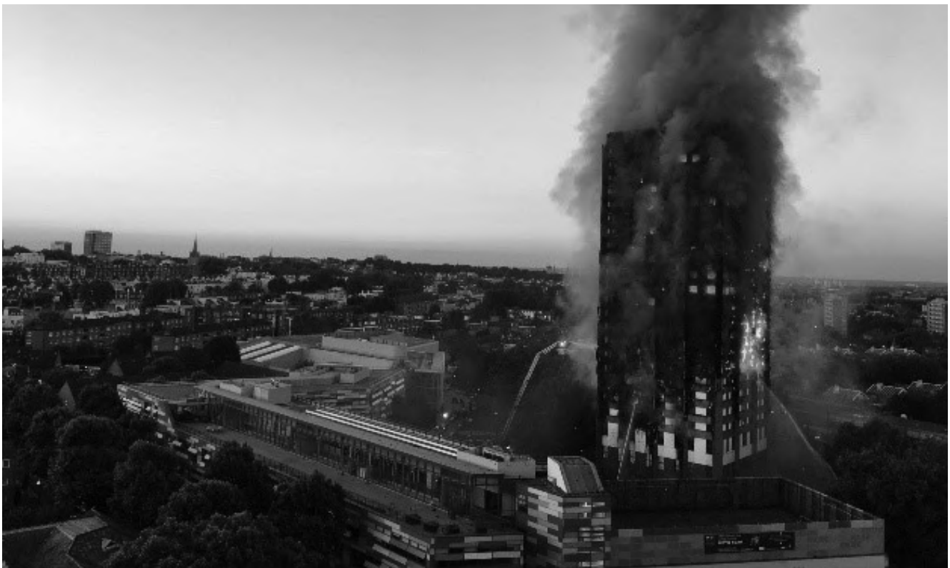
Figure 5. Fire at the Grenfell tower, London, 2017
