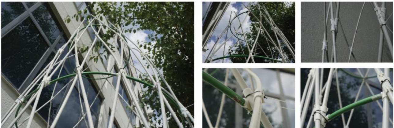
Figure 8 Assembly process of the PVC pipe structure and details photos: author and Sara Codarin
