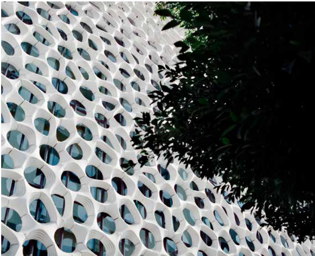
Fig. 6 – Torre de Especialidades, Hospital Manuel Gea Gonzales, elegant embellishments, Daniel Schwaag and Allison Dring (2013), Mexico City. The second skin module, realized in and coated with a titanium dioxide, performs a smart role in reducing air-pollution while daylight activated, acting at the same time as sun shading system; their specific design non repetitive and inspired by fractals, obtained with thermoformed plastics, contributes to the maximization of their effect.
