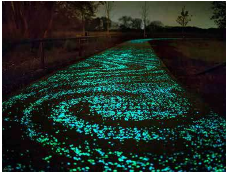
Fig. 4 – Fluorescent concrete employed in a cycling path in place of a traditional lighting system. El excelsior ph. Source: https://www.uniglowproducts.com/glow-in-the-dark-concrete-and-cement/
