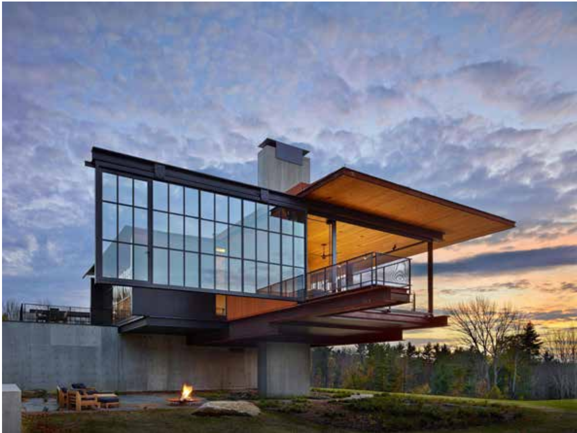
Fig. 5 – Berkshire Residence, Olson Kundig (2014), Berkshire, Massachusetts (USA). Private residence designed as low-tech smart home, symbolic of the smart definition given in the contribute. In this project indeed, facades are able to transform without recurring to advanced technologies but just by means of a complex system of cranks and levers. Benjamin Benschneider ph. Source: https://www.olsonkundig.com/projects/berkshire-residence/
