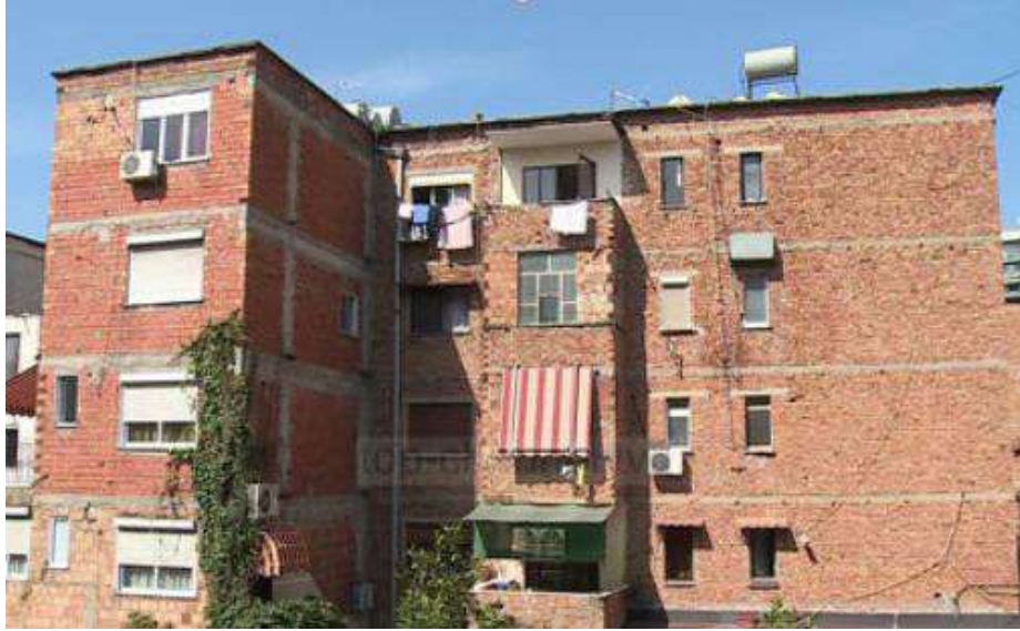
Fig. 4: The reference building
