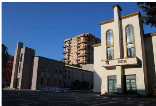
Fig. 1: National Theater of Albania, before demolition. Author: Doriana Musaj
