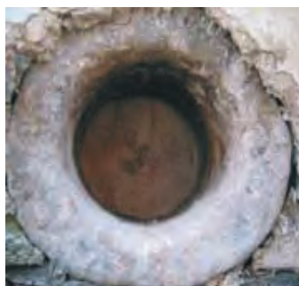
What is this? This stone niche in the wall was partly covered by many layers of plaster.
