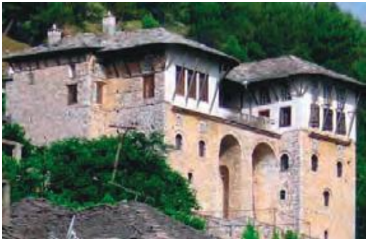
Gjirokastrian residential building
