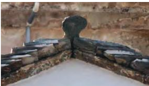
Stone roof detail
