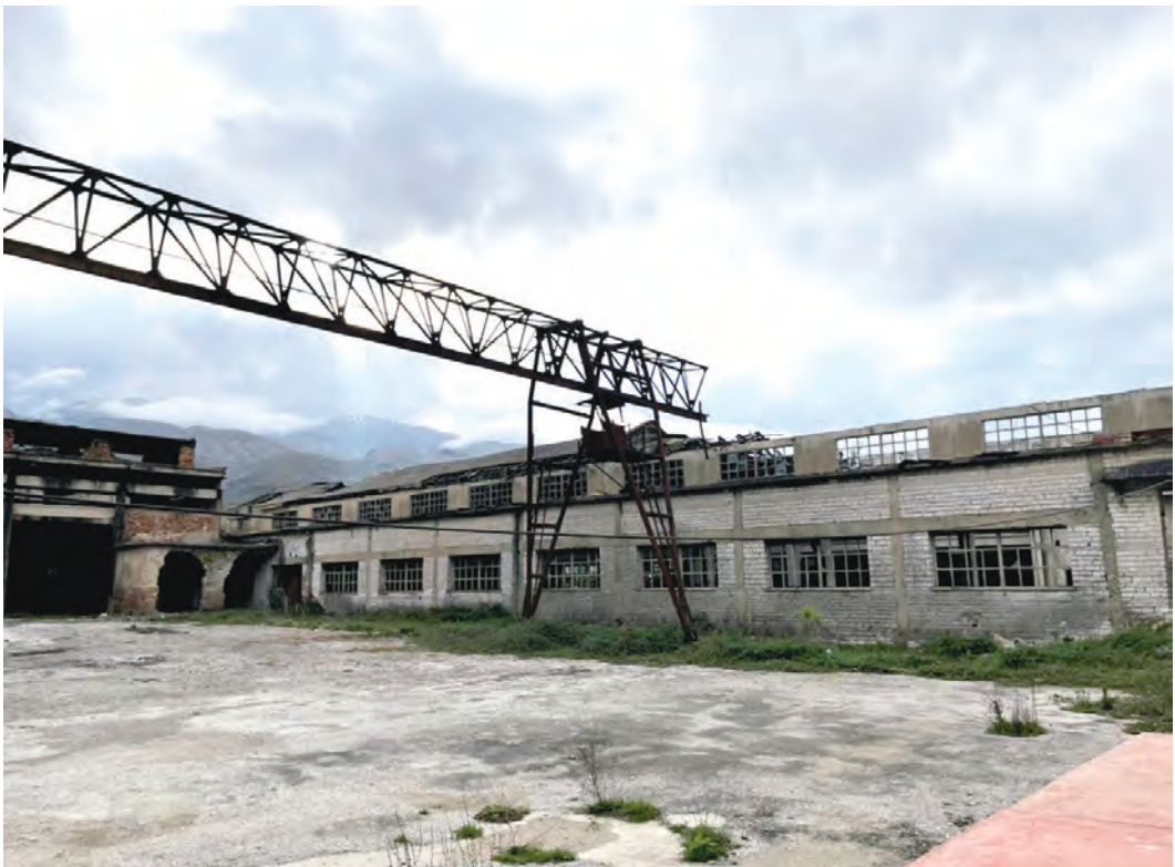
Fig.1 / Existing situation of Metal Plant, Gjirokastra, . Source / the author.
