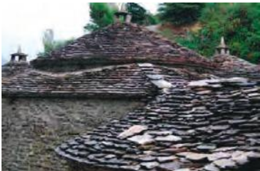
Stone roof of the Hamam
