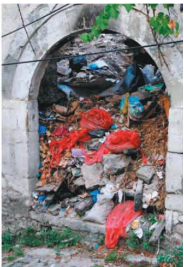
Ruin filled with garbage
