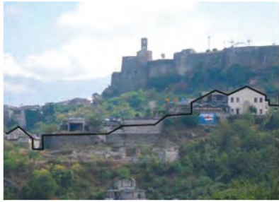
The concrete deck of Fantazia Area can usefully be demolished.
