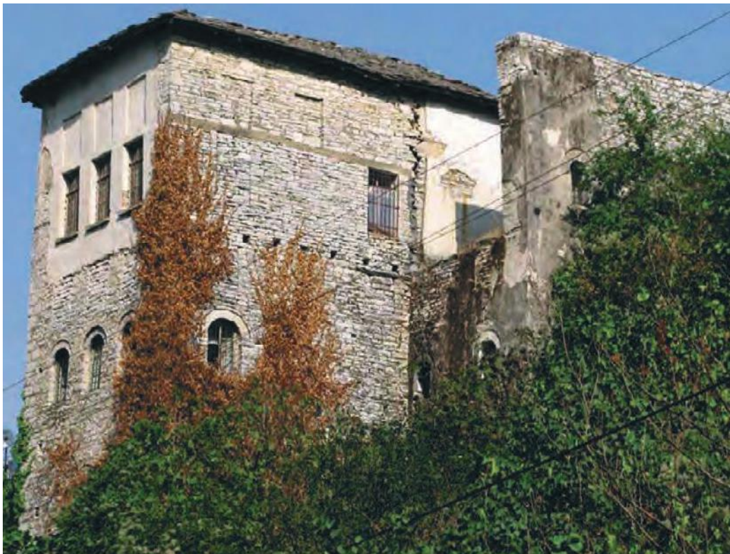
A common view in Gjirokastra, the impressive walls of cut limestone with symmetrical windows and heavy stone roof. Photographer: Elsa Notstrand
