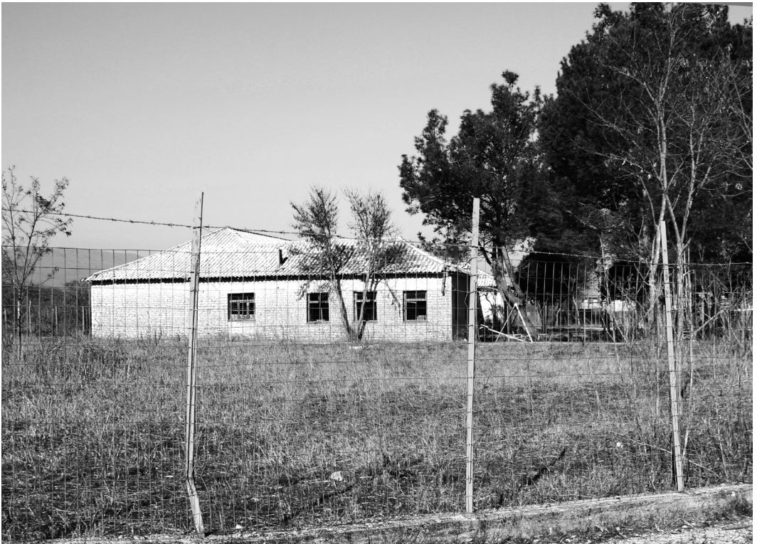
Fig.6 / School conditions. Deterioration of public spaces. Source / the author
