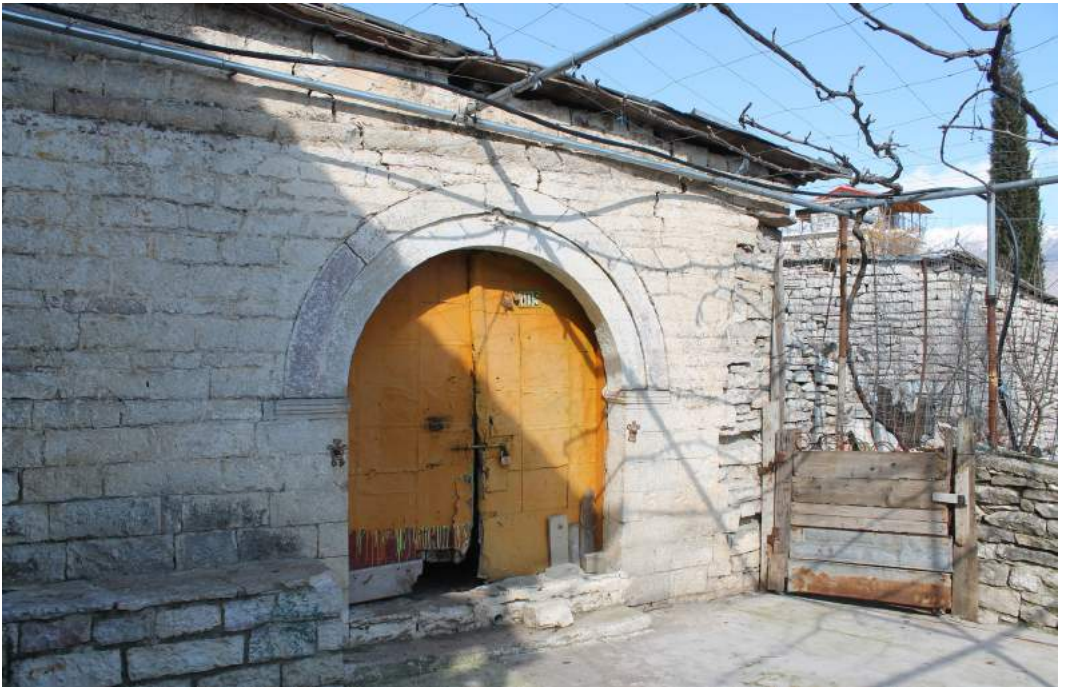
Fig.1 / Typical entrance of stone house in Jorgucat. Source / the author
