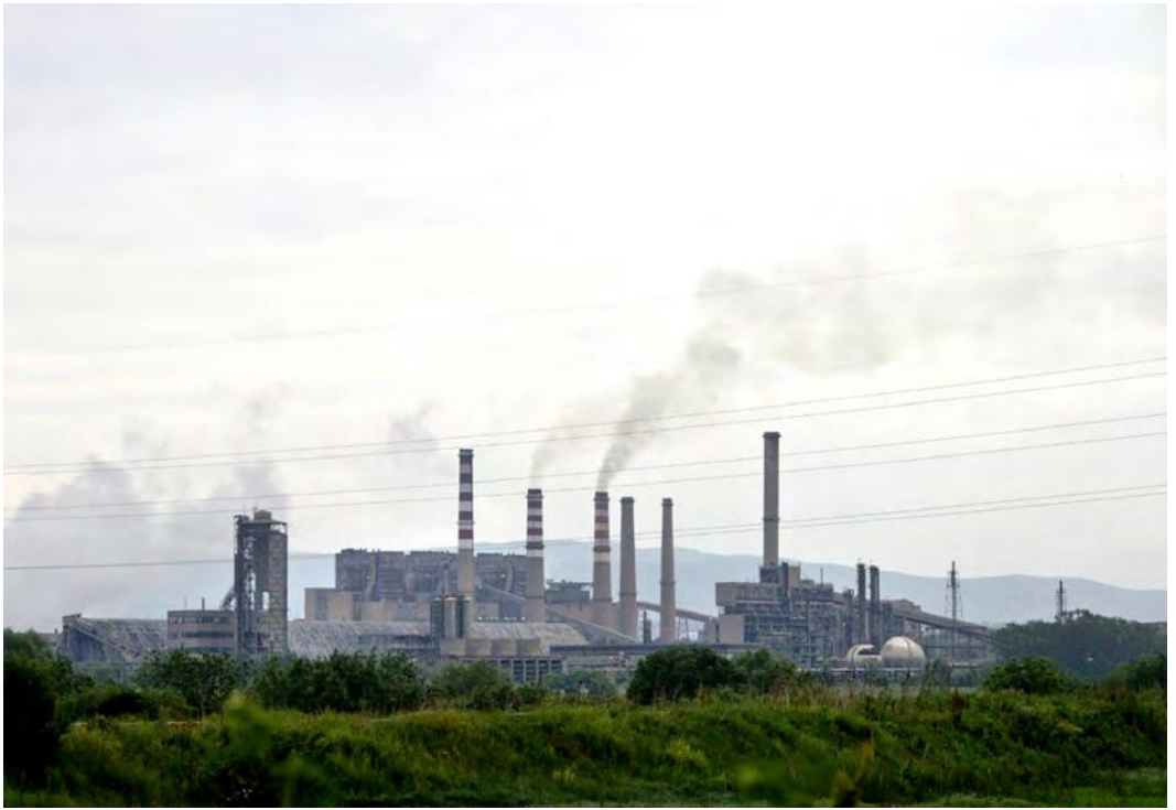
Fig5 / Coal-fired power plant, Prishtina. Source / Visar Kryeziu, International Consortium of Investigative Journalists. 2015.
