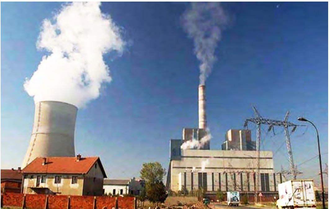
Fig1 / Obiliq Power Plant Source / www.insajderi.com
