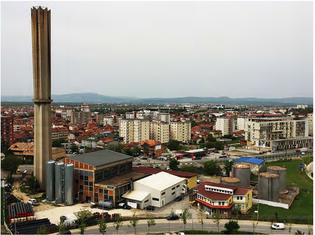
Fig2 / Termokos main building Source/ termokos.org
