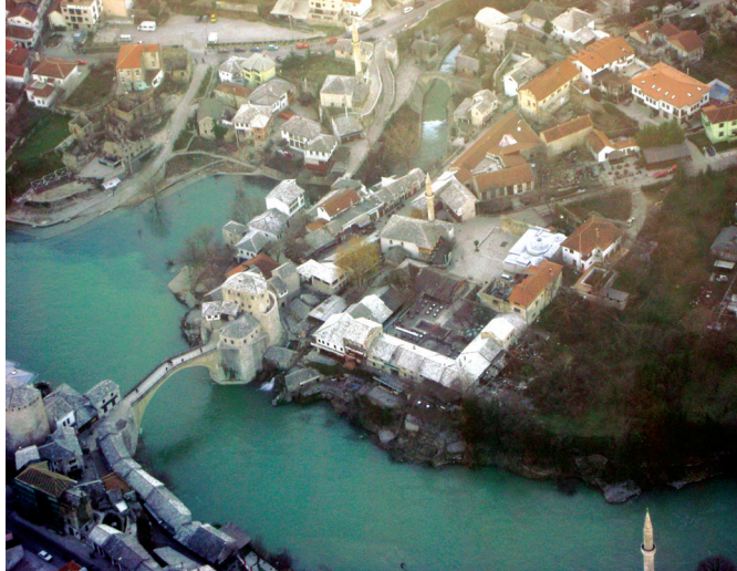
Fig. 12 –Aerial view of the bridge
