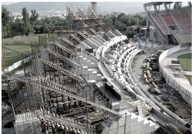
Fig. 31-32 – The Philip II Arena during construction
