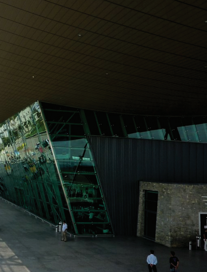
Fig. 6 - Picture of Tirana International Airport "Nene Tereza" taken from the bus station
