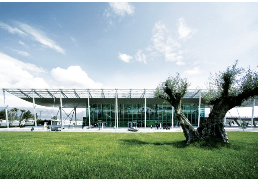
Fig. 5 - Frontal view of Tirana International Airport "Nene Tereza"
