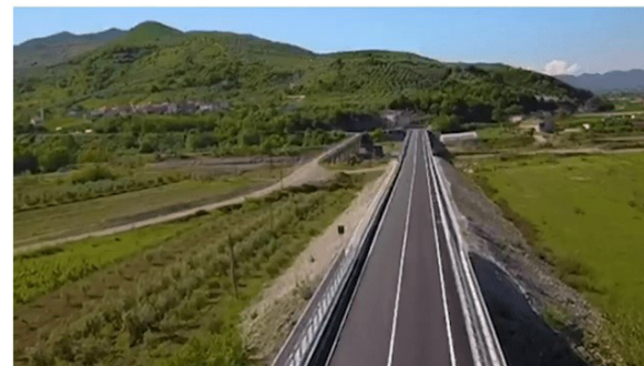
Figura 7. Aksi rrugor Elbasan-Banjë [https://elbasaniflash.al/video-elbasan-banje-rruga-me-infrastruktura-me-te-mire-per-banoret-dhe-vizitoret/]
