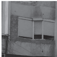
EXTRA SPACE-STORAGE AREA
