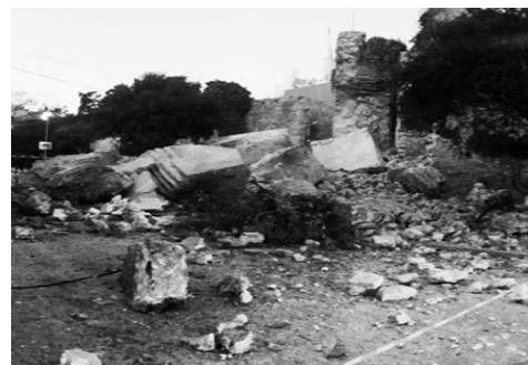
Figure 5. The Castle Tower of Durrës after earthquake/ source by the author
