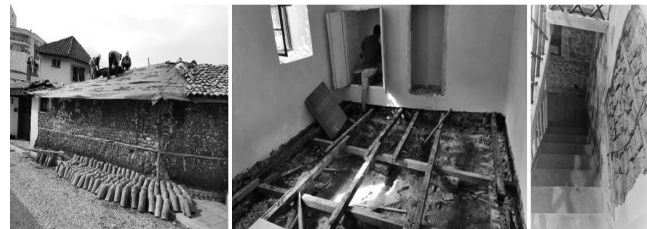
Figure 3 a,b,c. The use of adobe in the lowlands of central western Albania. View of the ground floor raised above the ground level. View of the inside house with perimeter walls in stone until 2m high and then the continuation is in adobe wall.
