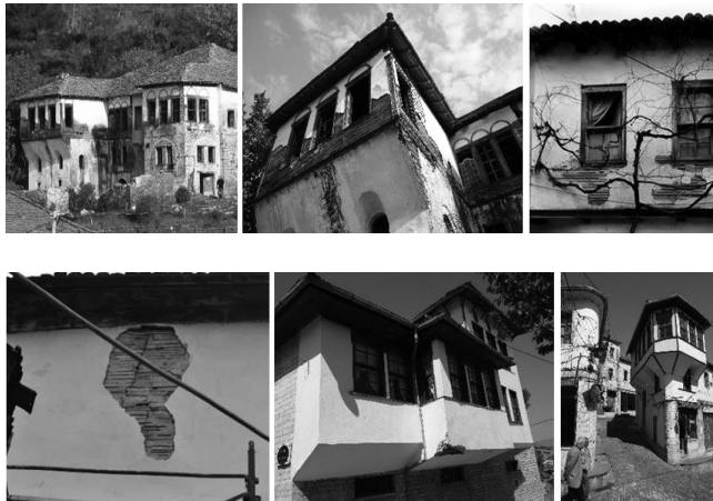
Figure 5. The use of adobe for the çatma technique in Berat e Gjirokastra rës Street and their transversal roads, or the eastern part along Elbasan road.
