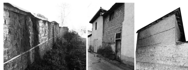
Figure 4. The use of adobe in Dibra area
