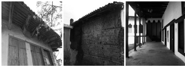
Figure 7 a,b,c. Protruding roof/Wood beams in the external walls/Porch space in front of the house
