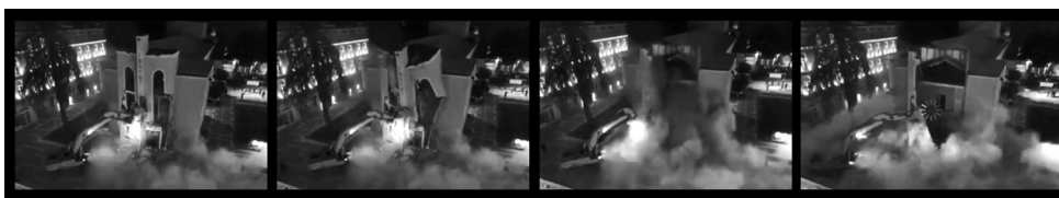
Figure 2. The destruction of the Theater. Source: Albanian media.
