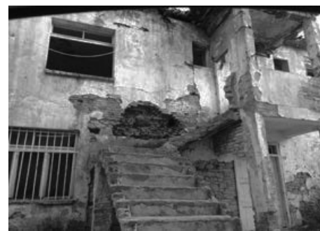
Figure 8. External Adobe walls of a traditional house in Kavaja, coated with an external brick layers
