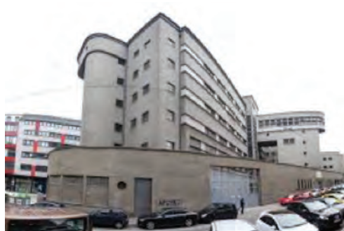
Fig. 22 (a-b). Electrical substation Favoriten, Vienna, outdoor and indoor views today
