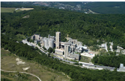
NEW Perlmooser Cement factory Built: 1894 / 1968 Function: Cement factory
