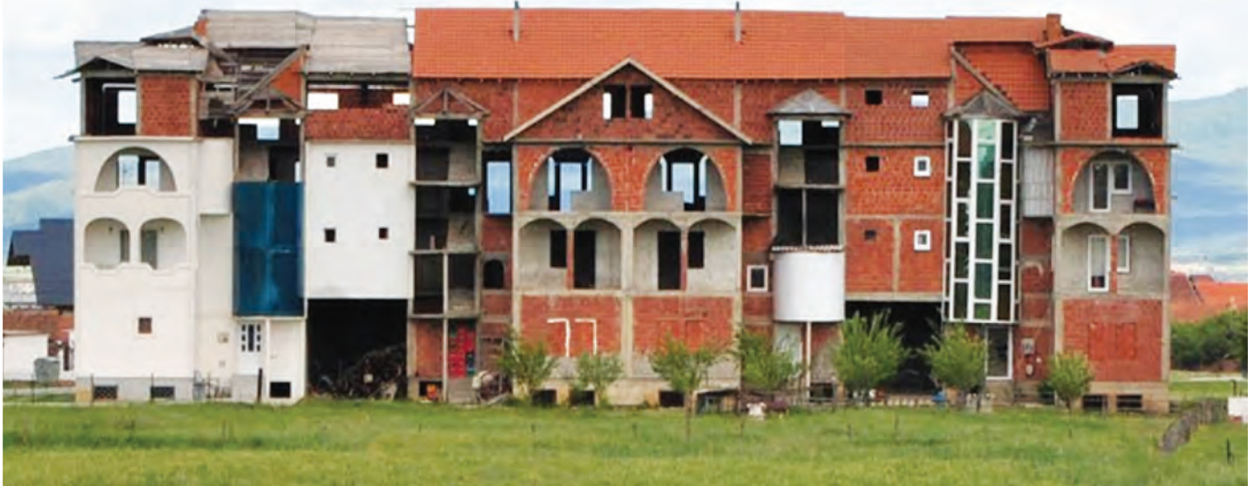
"Horrorchitecture", Lipjan, Kosovë (photo by A. Bajmaku 2013)
