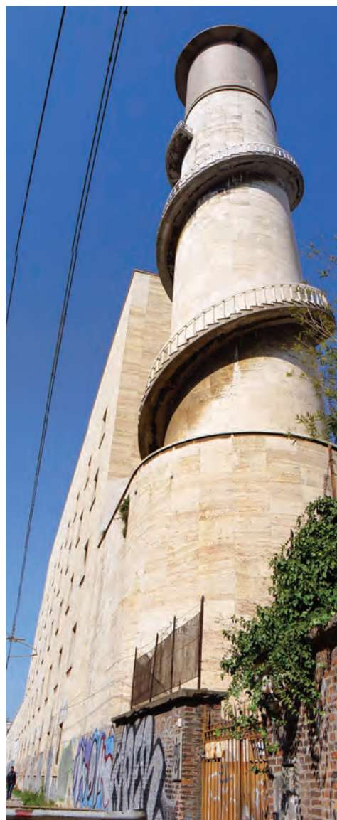
Fig. 13c Detail Station Termini in Rome by Angiolo Mazzoni.
