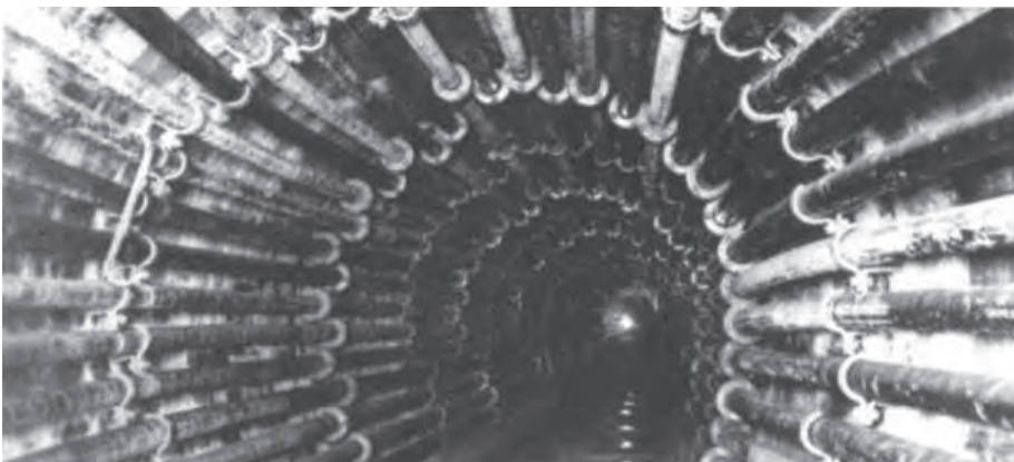
Fig. 17 Top: Historical Map: Pneumatic Mail Tube Network, Paris, 1967. Bottom: Sewers with the tubes from the Poste Pneumatique in Paris. Image caption from the Ignite/LA: Molly Wright Steenson - A Series of Tubes, EP 7.
