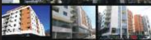
BRIDGE RESIDENTIAL COMPLEX, TIRANA
