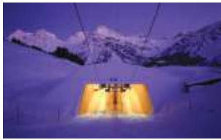
Bearth & Deplazes Architekten, [Carmenna Chairlift Stations, Arosa, 2001.] © Ralph Feiner
